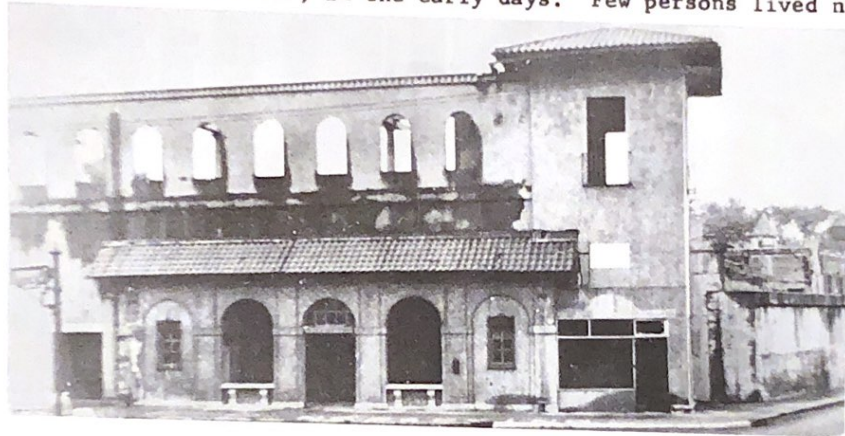
The empty shell of the once-attractive Chester Heights station became a decrepit eyesore after abandonment of the N.Y.,W.& B.
