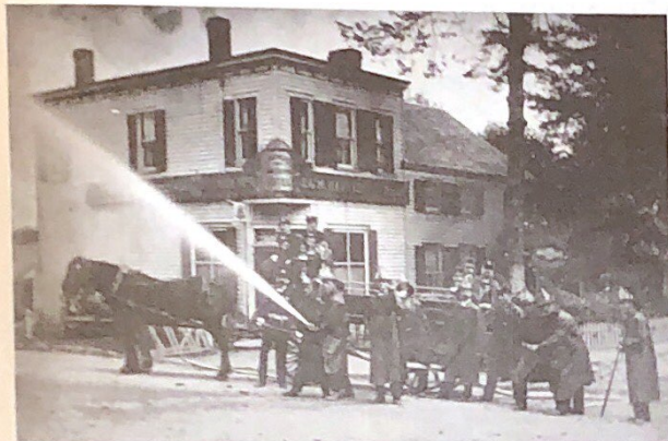
Union Corners Hose Company, trying out equipment in front of Fischer's Tavern, which was headquarters for the company for many years. Photo courtesy of Eastchester Historical Society.
